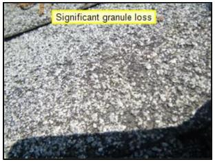
(2) One or more shingles or shingle tabs were missing or damaged at the front of home. A thorough evaluation of the roof and repair by a competent roofing contractor is recommended.
