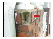
**1.13** The chimney has a weather cap but no spark arrestor, which is recommended but not required by any building standard. The lack of it will allow the entry of birds and animals into the chimney.
