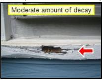
(2) Some of the wood framing around the attic windows was black, as if there may be a leak. The window was dry at the time of the inspection. We recommend an evaluation of them during a period of heavy or prolonged rain. Note that it may be due to an old leak that has been repaired.
