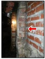
(2) The foundation footings have been undermined by trenching or soil excavation in one or more areas. An evaluation by a foundation specialist or structural engineer and repair as deemed necessary is recommended.
