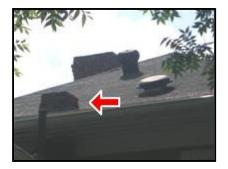
**2.5** (1) Every gutter downspout does not effectively discharge water 4 to 6 feet away from the house foundation. Although we rarely see it, we always recommend that downspout extensions be installed for the general welfare of the residence and its foundation.
