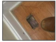
(2) The floor in the 1st level den has apparently dropped about one inch. We can elaborate, but you should consider an evaluation by a licensed general contractor or structural engineer.
