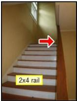
(5) The guardrail post at the top of the main stairs is not firm. Service is recommended to firmly attach the railing to the floor.
