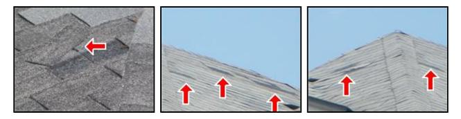
(3) A patched area of shingles was observed at the front of home. You should confirm that the repairs were performed by a competent roofing contractor.
