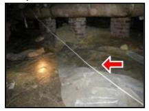
(10) Much of the original wiring and equipment has apparently been de-energized and replaced. However, most of it was left in place. Or recommendation is to remove all unnecessary wiring and equipment to eliminate any possibility of inadvertant energization.
