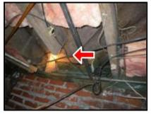
(4) A floor joist was split. An evaluation and repair as deemed necessary by a licensed contractor is recommended.
