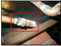
**5.1** (1) The visible portions of the drain pipes include an older cast-iron type, which are not as dependable as modern PVC drainpipes.
