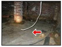
4 (9) In the crawl space, one or more electric cables was on the ground or dangled overhead. Electric cables
