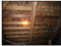
(2) A ceiling joist at the attic entrance has been cut and was not braced to compensate for the opening. Service by a licensed contractor is recommended.
