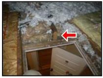
**7.6** Roof sheathing is water damaged around the chimney. Other areas had small portions that appeared to be water damaged. An active leak may exist and we recommend an evaluation and repair as deemed necessary by a competent roofing contractor unless the current owner can demonstrate that repairs have been performed. The areas were dry at the time of the inspection.
