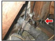
(4) Two open electrical junction box(s) were observed in the attic space which should be sealed to contain any arcing or sparking that might occur.
