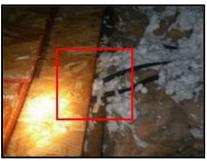
(6) No romex connector or strain relief bushing was provided to prevent a wire from making direct contact with the sharp edges of the junction box at the attic fan.
