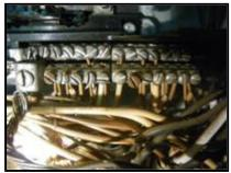
4) White conductors were used as ungrounded conductors (hot wires) at the main panel. This is a common
