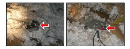
(5) Branch circuit wiring in the attic is susceptible to damage because it has been covered by floor decking. Abraded wires can be a shock or fire hazard. Service to re-route the wiring or remove the decking is recommended.
