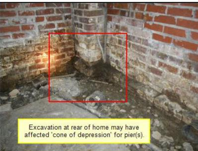
(3) Various portions of the floor structure was supported by various make-shift piers. Those floor supports exhibit poor workmanship are thought to be inadequate to provide permanent support to the floors. It is recommended that a competent and licensed general contractor or foundation specialist be consulted to provide a further evaluation of the adequacy of the floor supports and make necessary repairs.
