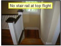
(4) The main stairs were not equipped with a standard, graspable, handrail. A standard handrail meeting today's standards is recommended for safety reasons. Information about proper stair railing and illustrations can be obtained here: www.aohomeinspection.com/pdf/IRC\_interpretation.pdf. (See page 10.)
