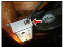
(7) There are unprotected electrical conductors within six feet of the attic access. Today's commonly accepted construction standards prohibit this practice and we recommend that they be relocated for safety reasons.
