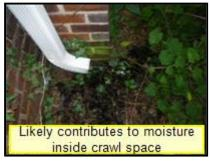
(2) The gutters and/or downspouts need to be cleaned and serviced to drain properly. The debris in gutters can also conceal rust, deterioration or leaks that are not visible until cleaned. Left unaddressed, clogged gutters will allow water to penetrate unintended areas and may result in decay to wood structures behind the gutters.
