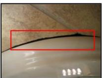
(2) There is a moisture stain on the library wall, which you should ask the sellers to explain or have explored further. The stain was dry at the time of the inspection. We could not confirm that repairs have been made.
