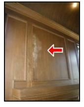
(3) There is a moisture stain on the 2nd level den wall, which you should ask the sellers to explain or have explored further. The stain was dry at the time of the inspection. We could not confirm that repairs have been
