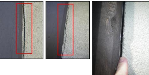
(4) There are large gaps at various locations where different wall materials meet. The wall structure and insulation was visible. Sealing the gaps to prevent water entry and structural damage is recommended. Note that we did not inspect behind the wall cladding and there is a possibility that structural damage may already exist to some degree.
