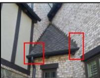
🔨 (2) Daylight can be seen around one of the chimney flues. Evidence of water entry into the attic was present (insulation that had been previously wet.) The flashing is apparently loose, incorrectly installed, or damaged. Service by a competent roofing contractor is recommended.
