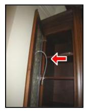
(2) The master bathroom custom shower contains a wood window, which we consider a poor design. Frequent maintenance will be necessary to prevent deterioration and decay. Replacement with a vinyl clad window is recommended.
