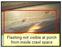
(2) The flashing for the side porch was sub-standard and may not be effective in preventing water entry against the house framing. The potential for water to penetrate behind the porch and siding may exist. We suggest that you have the installation method evaluated by a licensed general contractor.
