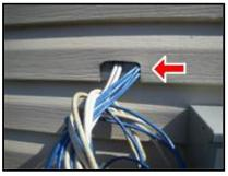
(3) The vinyl siding at the left side has one or more holes that may expose the sheathing to moisture. Repair or replacement of the affected sections is recommended.
