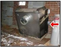
**4.4** (1) Large portions of the sub-floor are uninsulated. Insulating the sub-floor to a minimum level of R-19 is recommended for thermal efficiency.
