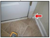
(2) We have detected a mold-like substance within the master bathroom closet and laundry room. You can learn more about mold from our web site <a href="here">here</a>. Note: our company has mold certifications from the International Association of Certified Indoor Air Consultants, and we can assist you with mold sampling and identification if you desire. Note: the amount of material was very small and no moisture was detected. A simple cleanup by a
