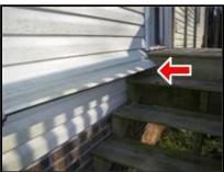
(2) A wall penetration near the electric meter were not adequately sealed. Service to seal the opening(s) is recommended. Failure to seal the opening could allow water to enter unintended areas.
