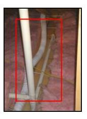
**7.4** Soffit vents have been obstructed by insulation. It is recommended that the insulation be sufficiently removed from soffit vents to provide adequate attic ventilation.
