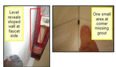
(5) The tile wall at the master bathroom appeared to be installed directly over sheetrock, and a cement wallboard base is called for to prevent water entry behind the tiles. If water enters behind the wall, structural damage may occur which may not reveal itself until years in the future. However, we cannot be certain of the construction method without destructive testing and you should therefore have it evaluated by a tile specialist or general contractor.
