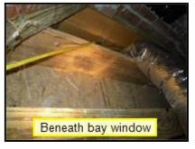
(2) Floor insulation has been installed up-side down. The vapor barrier should be installed against the subfloor. Service to reverse the insulation is recommended. And since the improper installation of insulation can trap moisture against the floor framing and may result in decay, the floor structure should be thoroughly evaluated by a licensed contractor.
