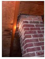
A large area of roof sheathing was noticeably different in tint (darker colored) at rear of house which may indicate moisture intrusion. Area was toward kitchen. Moisture meter did not detect a higher than normal moisture content, but buyer may want to further investigate this area after a period of heavy rain (roof shingles above this area were also different in tint—lighter colored).
