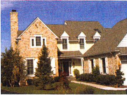
Photo 1 (left): Pennsylvania Stucco “Shack.” Eastern Pennsylvania is the stucco failure capital of the United States. Note the manufactured stone veneer—or lumpy stucco on the front façade. Photo 2 (center): Hardcoat Stucco. Three coats have been traditionally applied directly over a single layer of impregnated felt or asphalt-saturated kraft paper. Today, this results in a bond between the stucco rendering and the outer layer of the felt or paper, compromising drainage. Photo 3 (right): Manufactured Stone Veneer. Manufactured stone veneer claddings are similar to hardcoat stucco and perform in a similar manner. In a manufactured stone veneer, the outer coat of stucco is replaced with a thin stone layer.
