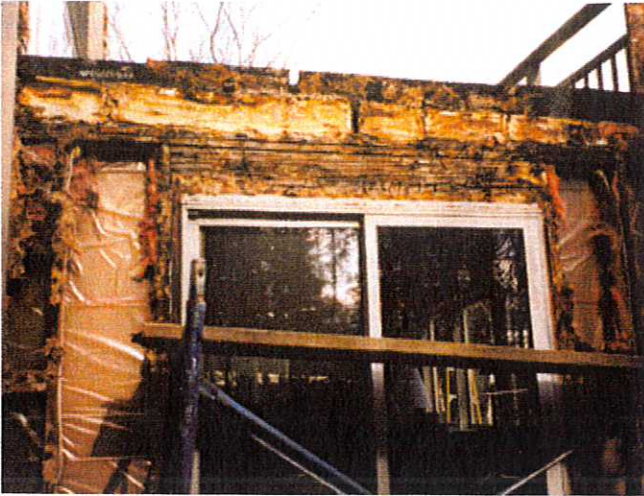
Photo 5 (left): Failure on Steroids. Note the plastic vapor barrier “accelerant” in this Vancouver, Canada, building. Photo 6 (right): Hard-coat Stucco Bonding to Plastic Building Paper. A young, happy engineer discovers stucco bonds to plastic building papers, preventing drainage. The engineer is my friend Chris Schumacher. May he remain this happy when he gets older.
