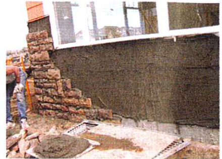
Photo 1 (left): Pennsylvania Stucco “Shack.” Eastern Pennsylvania is the stucco failure capital of the United States. Note the manufactured stone veneer—or lumpy stucco on the front façade. Photo 2 (center): Hardcoat Stucco. Three coats have been traditionally applied directly over a single layer of impregnated felt or asphalt-saturated kraft paper. Today, this results in a bond between the stucco rendering and the outer layer of the felt or paper, compromising drainage. Photo 3 (right): Manufactured Stone Veneer. Manufactured stone veneer claddings are similar to hardcoat stucco and perform in a similar manner. In a manufactured stone veneer, the outer coat of stucco is replaced with a thin stone layer.
