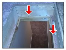
(4) No depth markers were evident in the attic space. Without insulation markers, the insulation installer cannot be assured that the proper level of insulation was provided. Service to install the marker and ensure that the proper amount of insulation was installed is recommended for thermal efficiency reasons.
