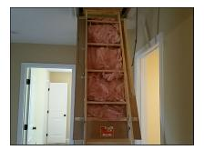
(3) Today's commonly accepted construction standards require foam sealant at penetrations into the building from unconditioned spaces or the outdoors. No foam sealant was provided at the attic entrance. Service by a competent person is recommended.
