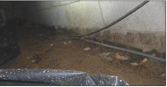
(3) Evidence suggests that the crawl space is not rodent or animal proof. Rodents have collapsable rib cages and can enter the home through small and narrow spaces. A competent person should ensure that the house is not accessible to rodents, snakes or other wildlife because they are a nuisance and health hazard.
