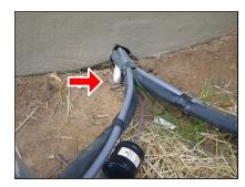
(3) The secondary condensate port was not plumbed to the drain pan. As a result, when the primary drain line becomes clogged, the condensate inside the air handler has no path to escape. It will rise in the air handler cabinet
