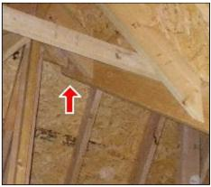
(2) Guardrails for personnel protection while on the attic deck were not provided. They normally are present. It appears the project was started but not finished. We recommend guardrails for safety reasons.
